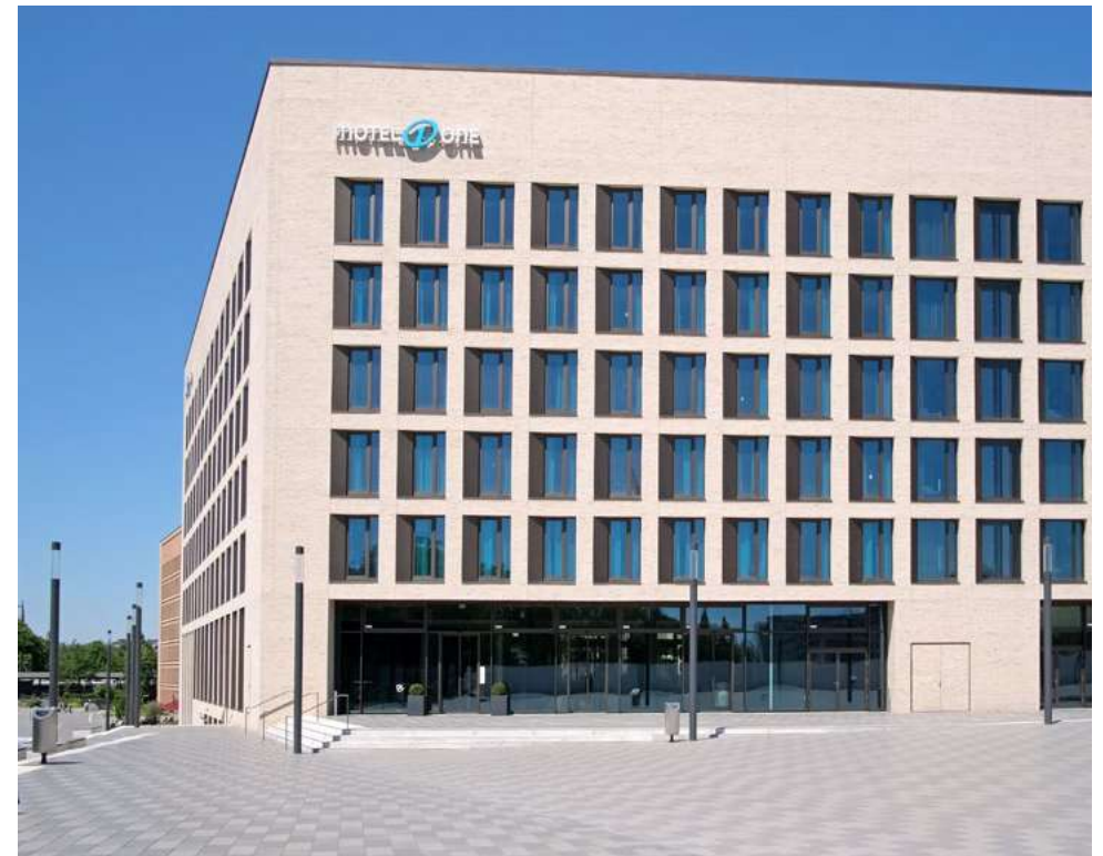
The hotel ensemble Southern Cross is part of the large-scale project MesseCity.
